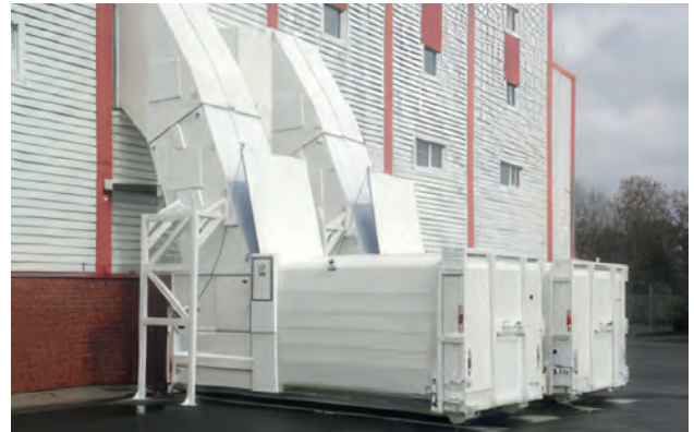
Wall connection feed opening from upper floor
